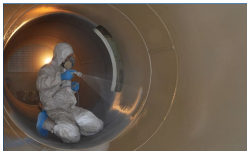
Spray applied Belzona lining
