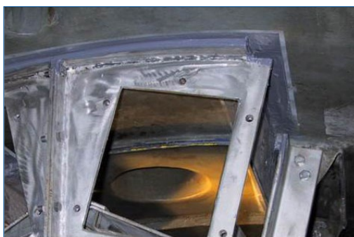
Overhead fittings bonded
